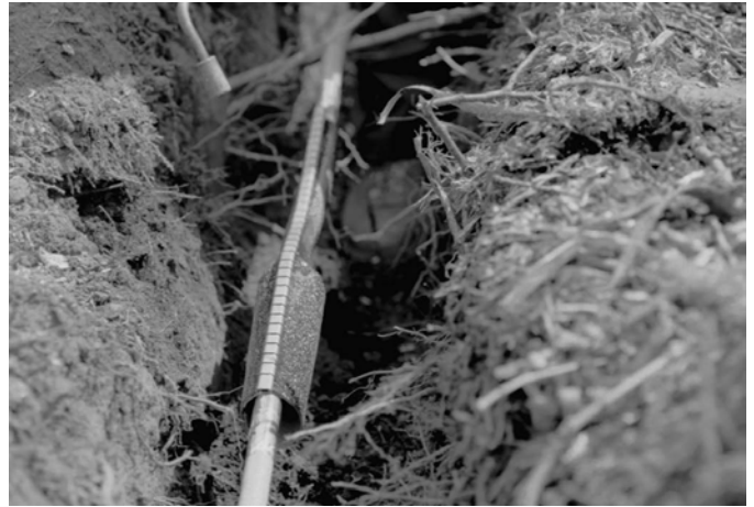
The CWST sleeve is simply wrapped around the damaged cable area and shrunk with a standard joiner's torch.
